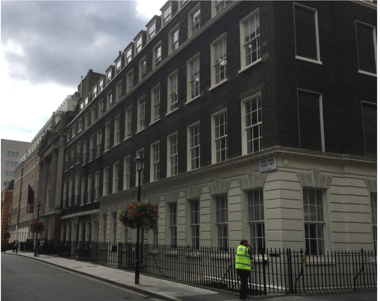
Wider view of the site from the corner with Adam Street
